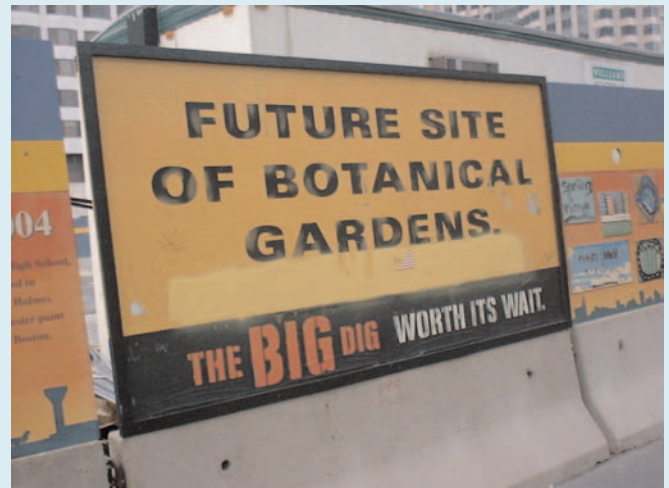
Big Dig in Progress 2002
