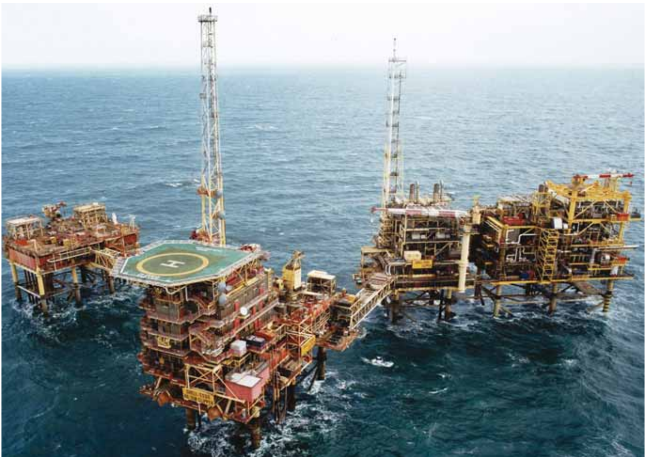
A typical North Sea Oil Rig
